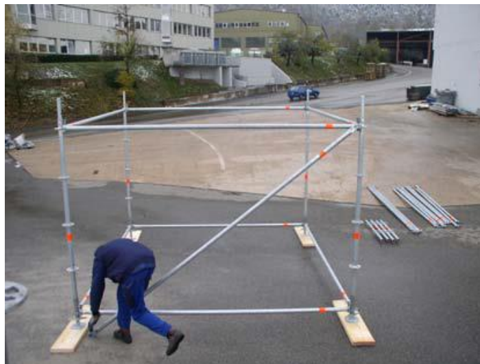
Fig. 4. Assembly of the first horizontal frame
